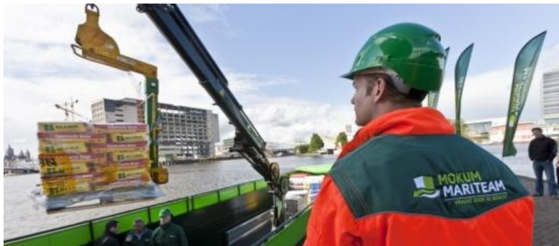
Figure 12: The City Supplier transhipping construction materials using its on-board crane (source: Mokum Mariteam)
