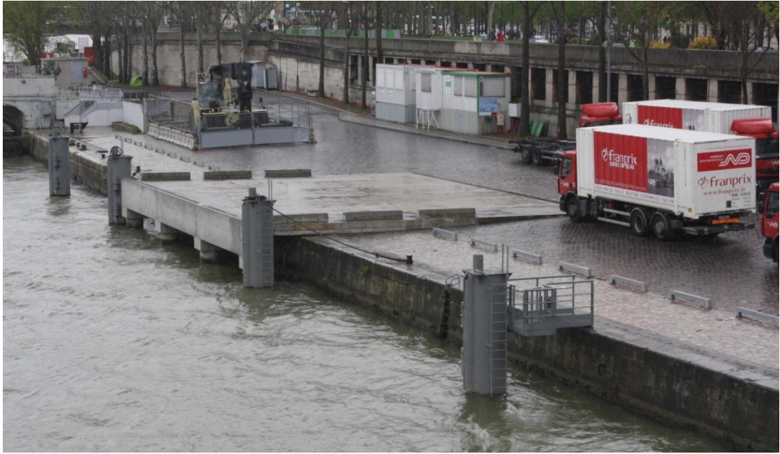
Figure 35: Port de la Bourdonnais – Paris – view of the reinforced quay wall (source: Technum)
