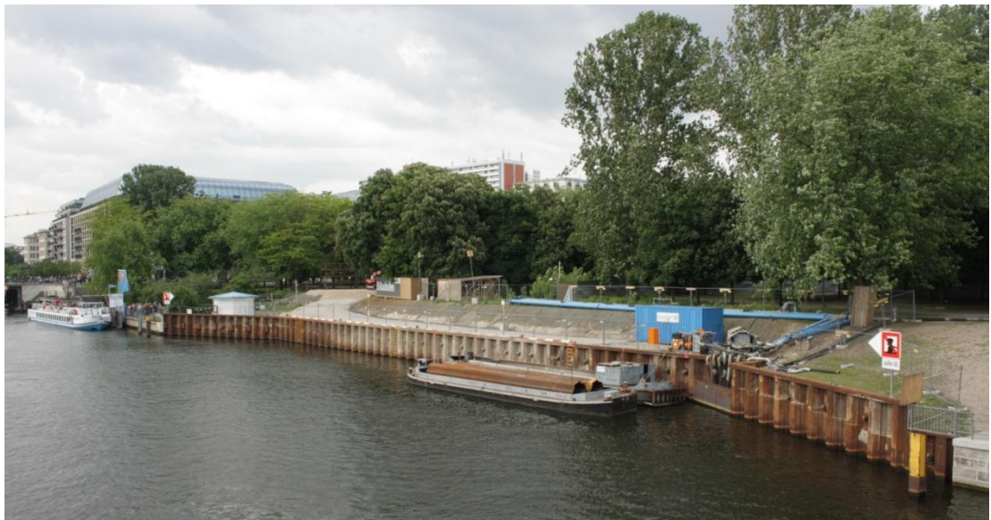
Figure 7: View from the other end of the platform (source: Technum)
