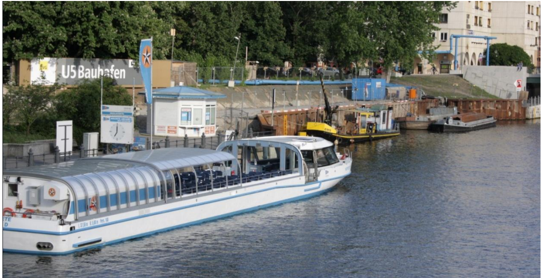
Figure 6: The new quayside on the River Spree, in the historic heart of Berlin (source: Technum)
